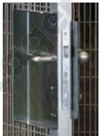
Door with approved panic lock. A door with panic lock can always be opened from the inside even when it is locked. Not working for sliding doors.
