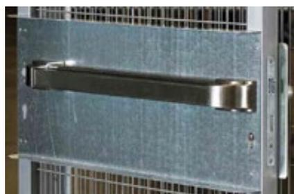
Door with approved panic bar and lock. A door with panic bar can always be opened from the inside even if it is locked. Not working for sliding doors.
